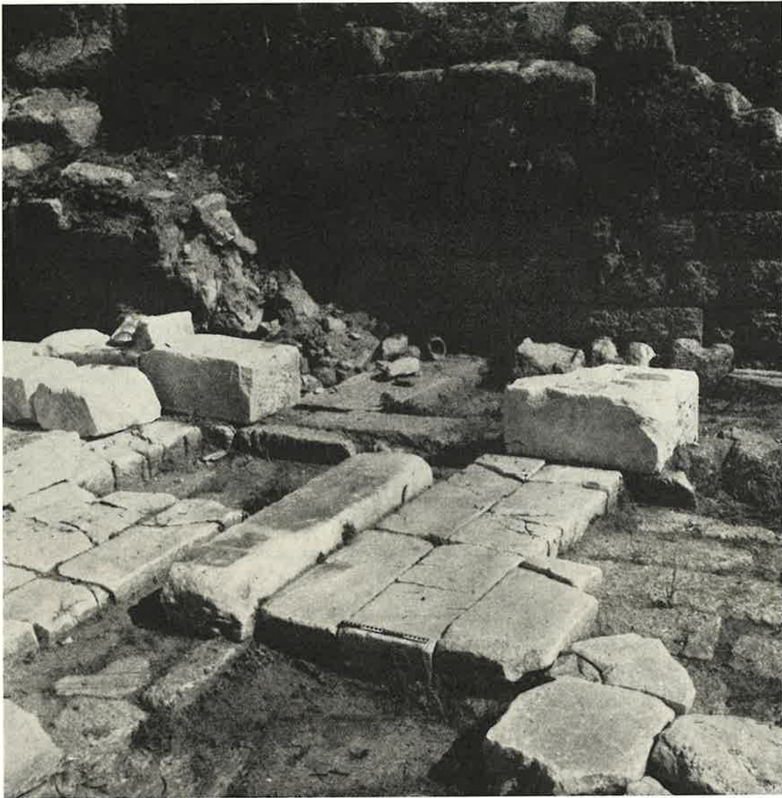
Fig. 20. Foundation of the East Propylaea, with the sill block H 31 and the orthostate block H 60 almost in situ (phot. Lingheim).
