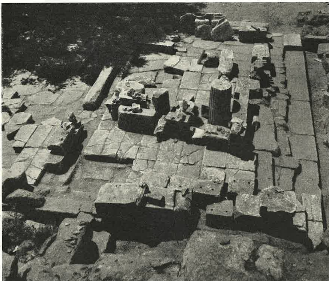
Fig. 19. Foundation of the East Propylaea viewed from the north (phot. Nilsson).
